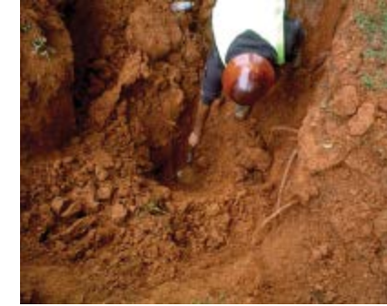
Using an acoustic detection pick-up stick.
