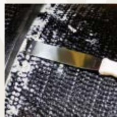
Insert tool between bell and spigot
