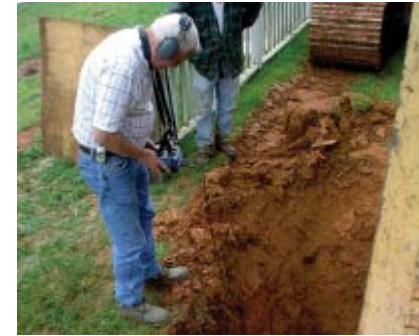
A Leak Detection Specialist uses acoustic detection.
