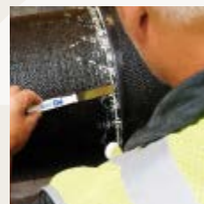
Check joints at various locations
