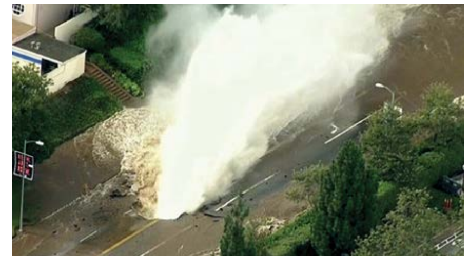
A water main break spews potable water.
